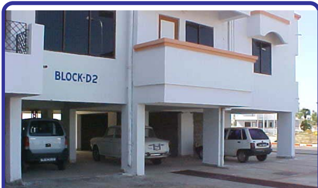
Figure 1: Ground storeys of reinforced concrete buildings are left open to facilitate parking – this is common in urban areas in India.
